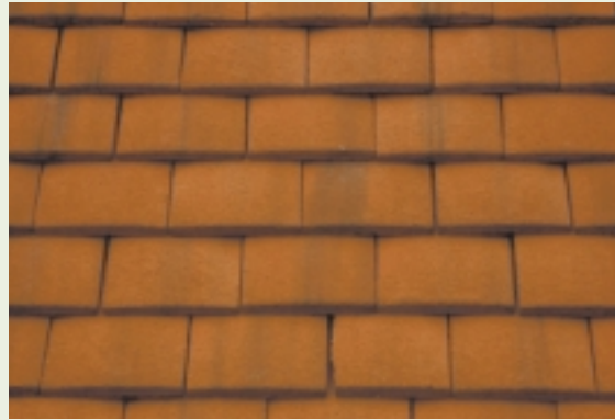
Orange/red hues are in keeping with the clay tiles traditionally used in the Surrey Hills, derived from the Wealden clay. Tile hanging, particularly to upper floors over brick or render construction, is a traditional feature.
