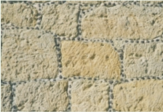
Bargate stone is a hard, coarse grained, calcareous sandstone, coloured by iron oxide. It is the main building stone in the area but is no longer quarried, so the best possible match should be used.
