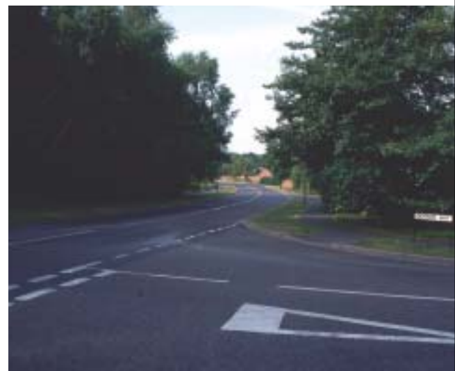
Goldsworth Park, Woking – Design requirements of roads have dominated
