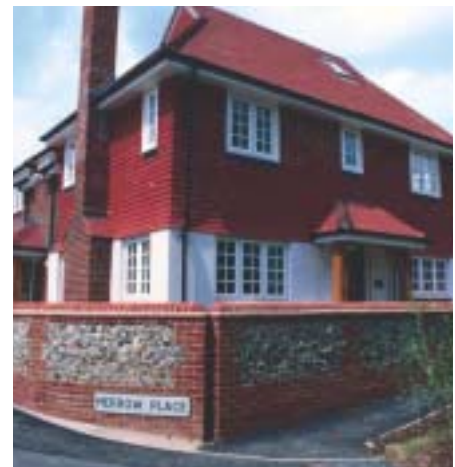
Merrow Place, Guildford Appropriate use of flint on boundary walls. Often the material of boundary walls can be a practical and appropriate way to mirror the local vernacular
