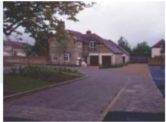
Caterham-on-the-Hill, Caterham Here an engineering solution dominates (speed control bend with forward visibility) to control speed rather than junctions and buildings
