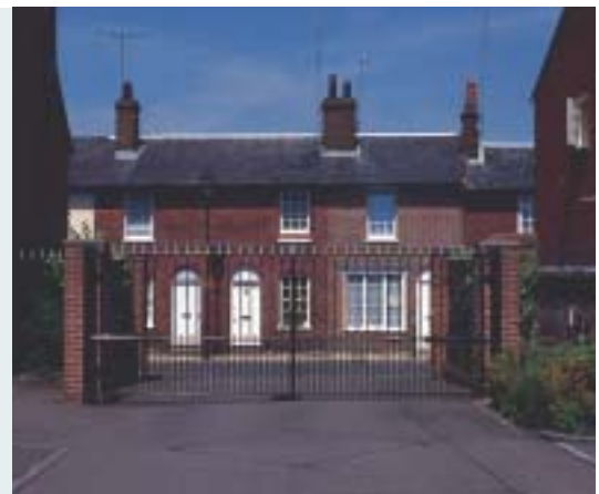
Central Dorking Gated estates – Provide internal security but do little to promote wider feelings of safety and community or enable pedestrian links with the surrounding area
