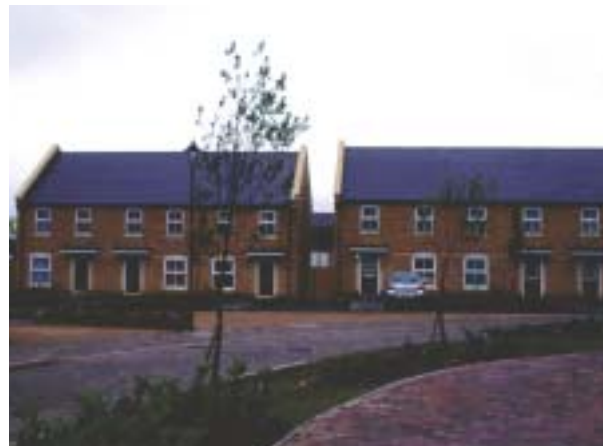
Caterham-on-the-Hill, Caterham Affordable housing and market housing side by side
