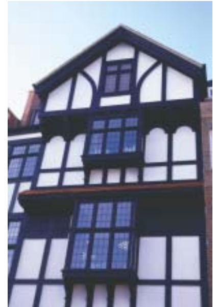
Timber framing – Charter Quay, Kingston upon Thames used in a convincing way on a new building
