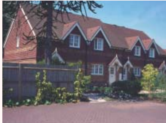
Stacey's Place, Elstead Village New development in Elstead based on the Village Design Statement
