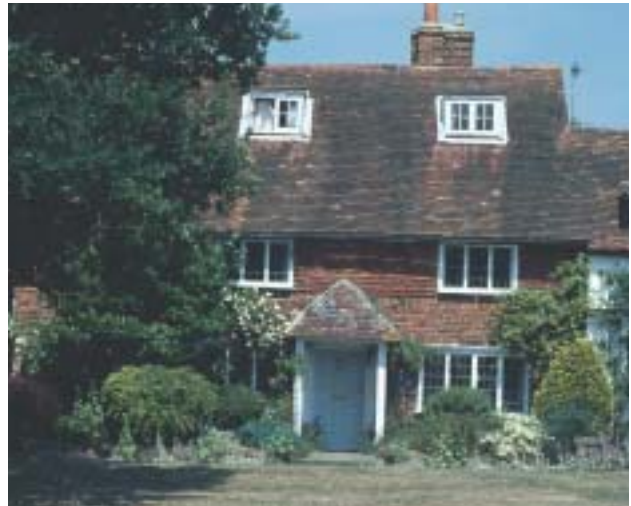
Brockham Traditional simple rectangular form with tile hanging, brick and clay tiles
