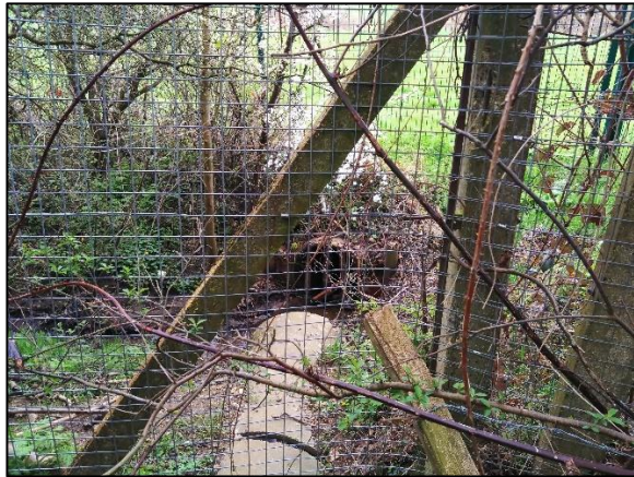
Photo 9 Culvert in east of site
