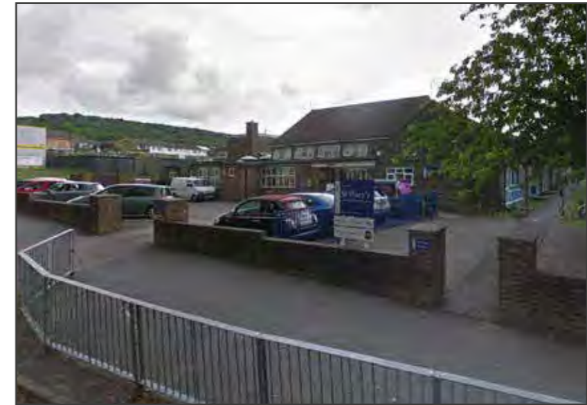
FIGURE 2.4: ST MARY'S C OF E PRIMARY SCHOOL - 2 MINUTE WALK FROM THE SITE
