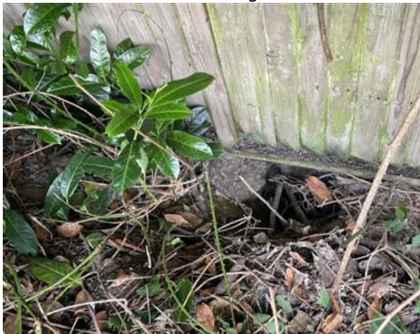
Photo 3 Hole 2, under fence
