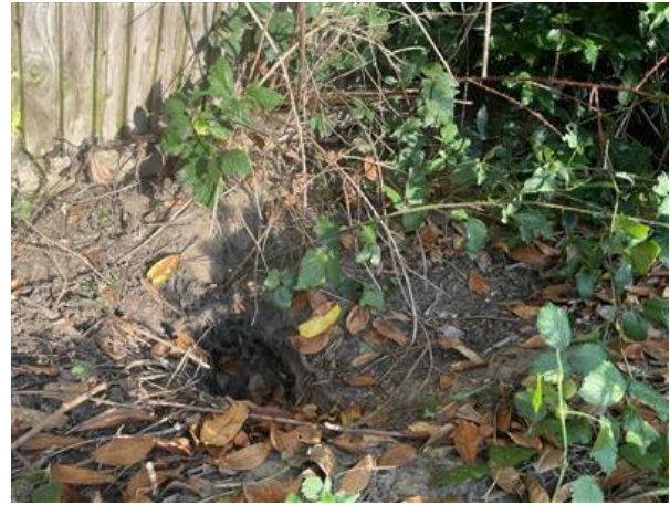
Photo 2 Hole 1 in proximity to the fence
