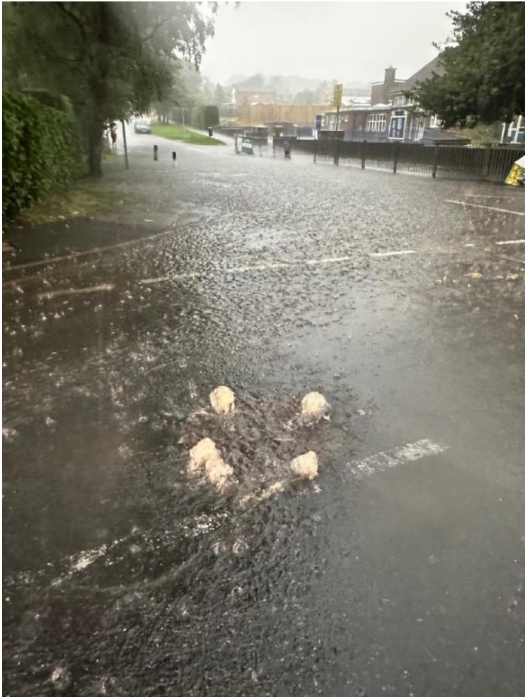
The existing 400-525mm surface water drain, flooding the Chichele/Silkham Junction August 2024. St Mary's School can be seen on the right.
