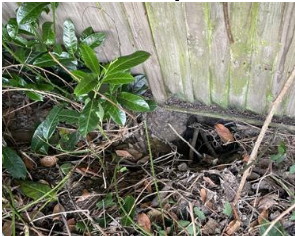
Photo 3 Hole 2, under fence
